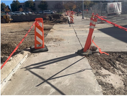
Example of obstructed pathway due to construction and also significant inclines without handrail.
